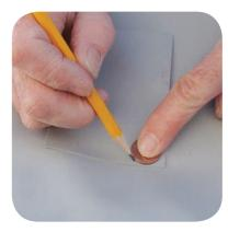
Using a pencil or ballpoint pen, trace the outline of the patch which should be large enough to overlap the damaged area by approximately 1/2". Angle the pen inward a bit so that the ink will be covered by the patch later.
